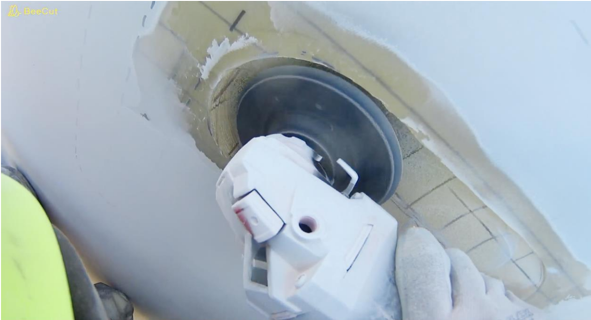
In-situ repair may release more micro plastics into the environment than the natural erosion itself.
